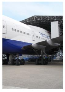
The free-standing scaffold structure was held in place by  $120 \times 1$ -tonne bags of 75/45mm stones and erected using tube & fitting scaffold with a Cassette Roof System. Tec-bolts were used to secure the internal and external sheeting.
