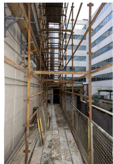
Rear of building (East elevation)
